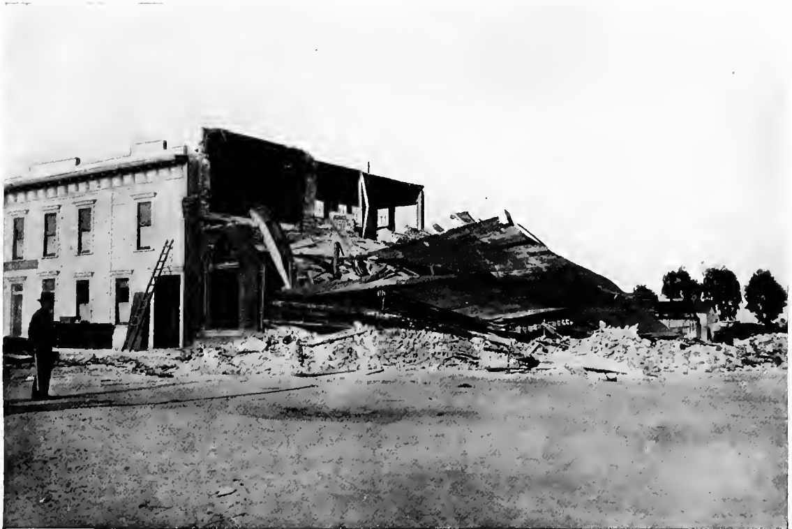
B. Wreck of 2-story brick building, San Mateo. Per J. C. B.
